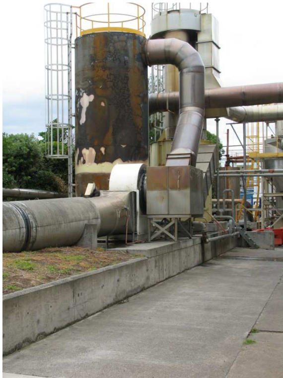
Fig 2: Humidifier/Scrubber Tower
